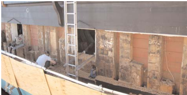
Portion of Constellation's Topsides Removed for Repair, Replacement
