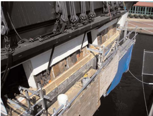
USS Constellation Hull Repair in Progress, Starboard Side
