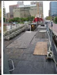
Above: USS Torsk , ca. 1945. Far left: view under the deck showing steel wastage. Left: view showing foredeck under repair today.
