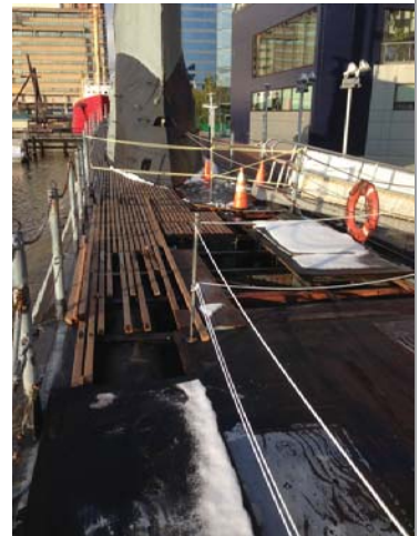
Looking forward towards the "sail". We are working aft from here.
