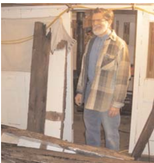
Volunteer Fran Marinaro surveys the demolition of the Midshipmen Quarters Deck.
